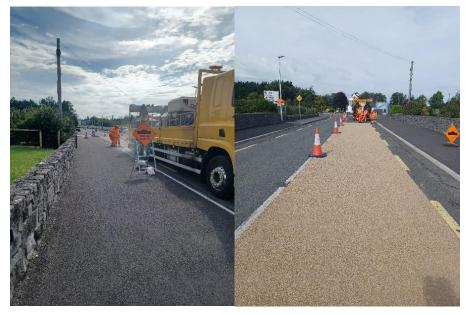
CAHERLISTRANE, INSTALLATION OF ANTI-SKID AND LINE MARKING AT NEW PEDESTRIAN CROSSING AT GAA GROUNDS.
